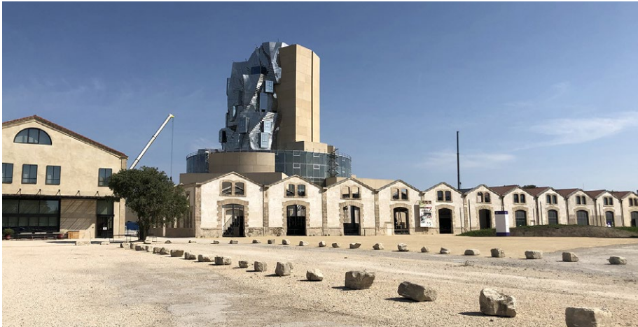
Figure 2. View of the LUMA Tower under construction.
